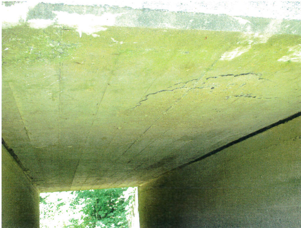
The underside of the structure
