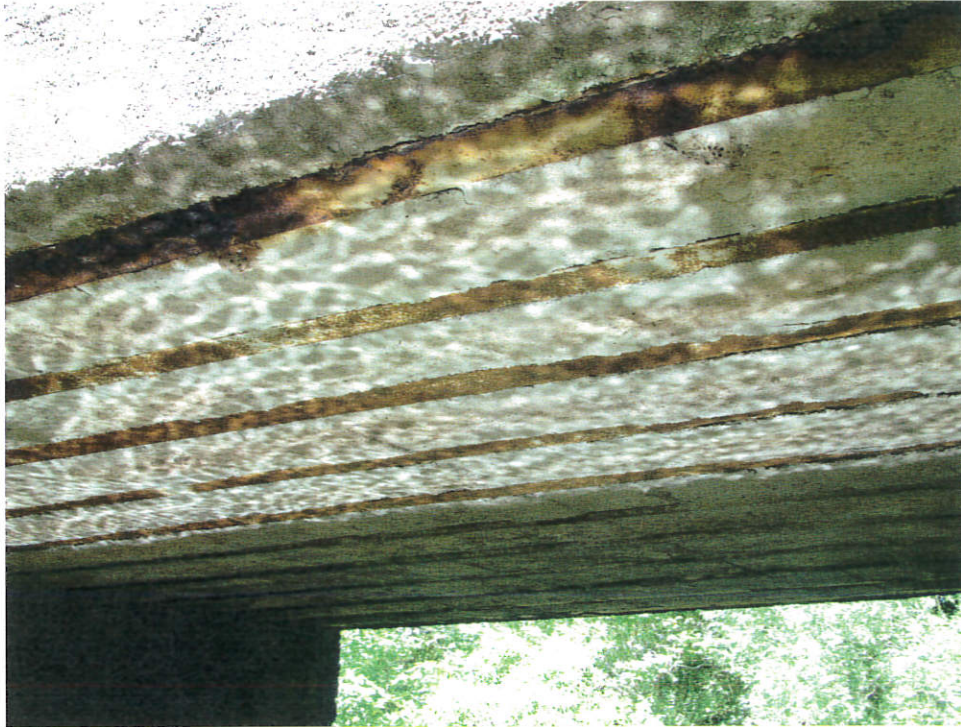
The underside of the structure
