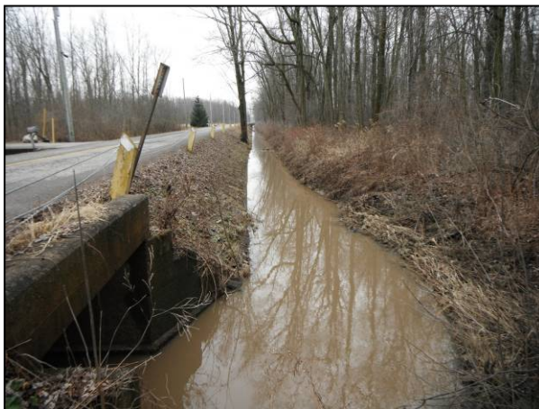
Photo 50: Reach 8-B, channel adjacent to White
