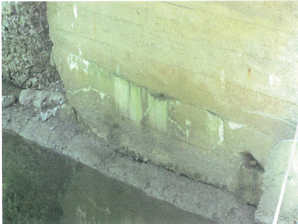
The east wall of the structure
