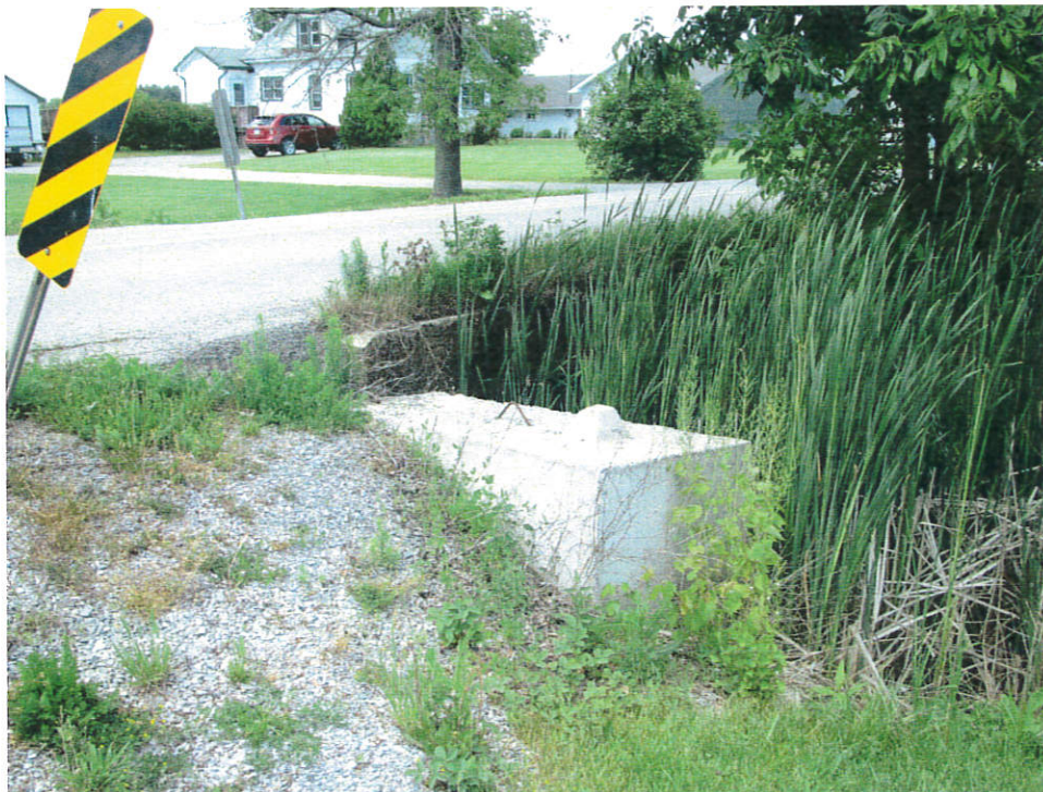
The east end of the structure
