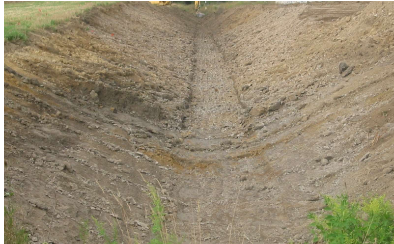
Figure 11 Trapezoidal Ditching Under Construction
