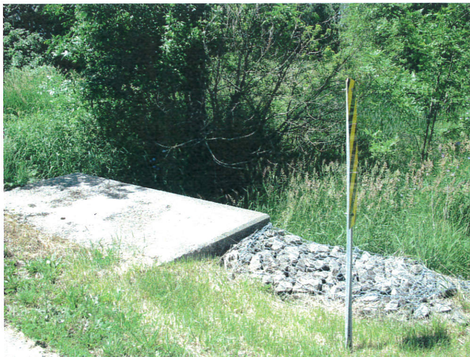
The west end of the structure
