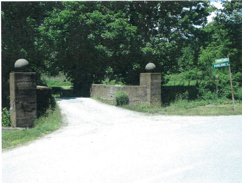
Roadway over the structure - Looking west
