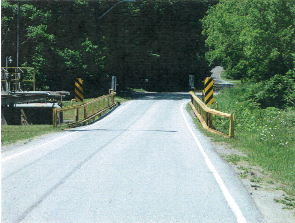
Roadway over the structure - Looking west
