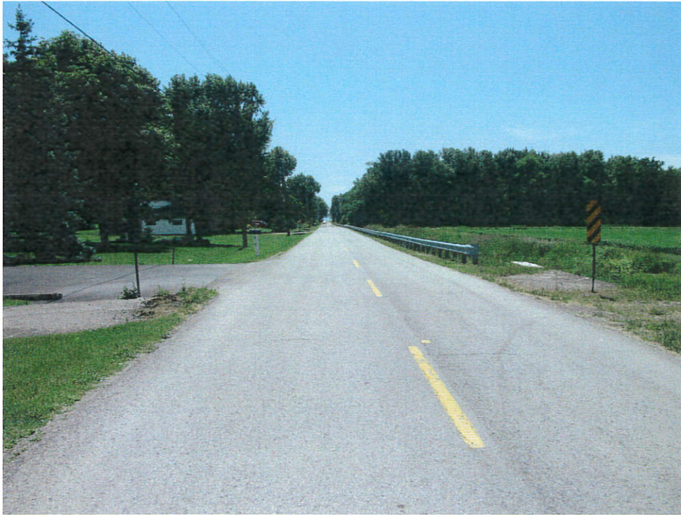
Roadway over the structure - Looking south
