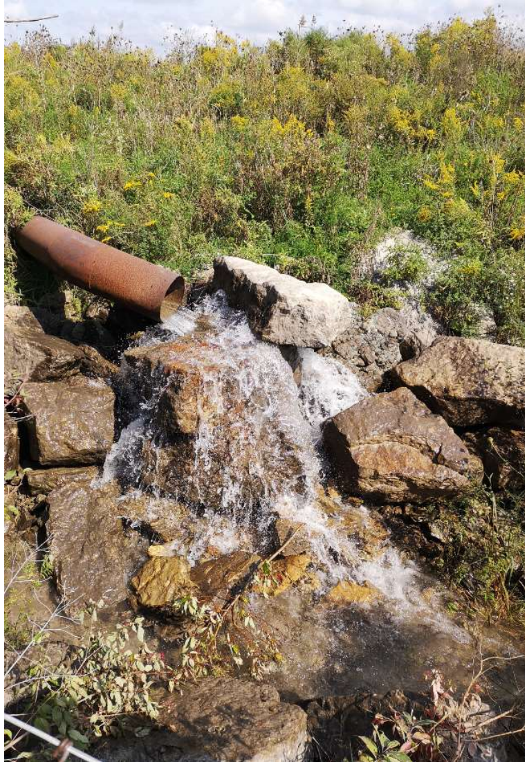
Figure 24 West Side PC Quarry Pump Discharge - Sept 19
