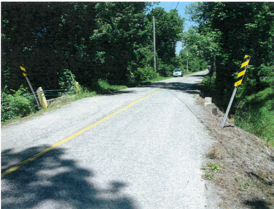
Roadway over the structure - Looking north
