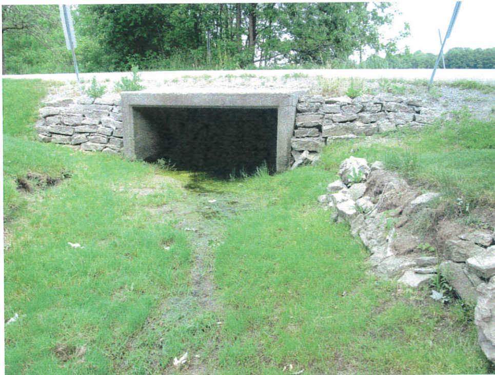
The west end of the structure
