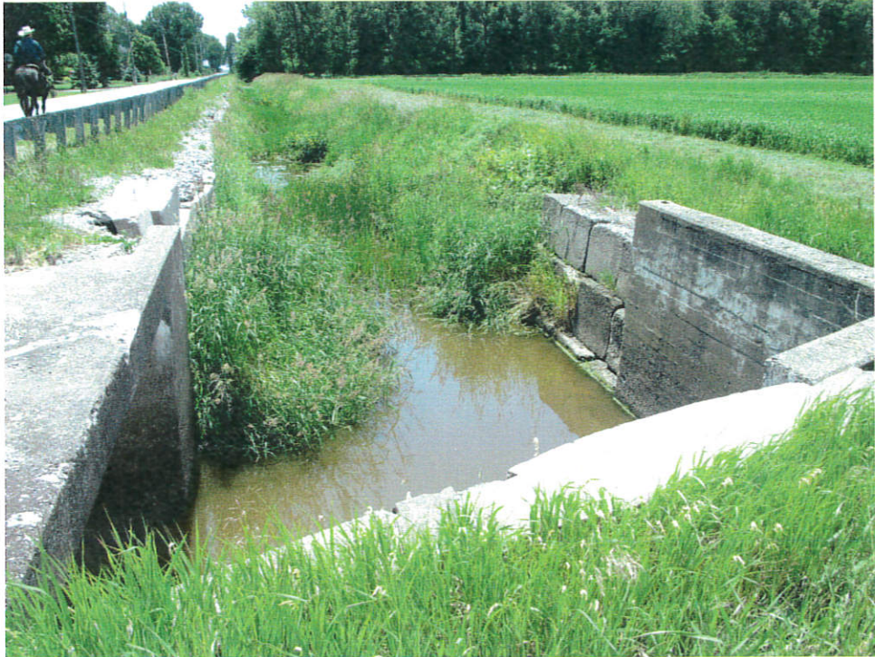
The west end of the structure
