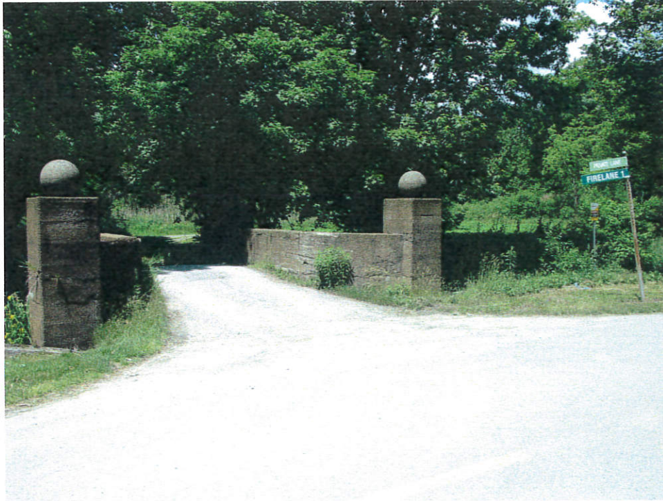
Roadway over the structure - Looking west
