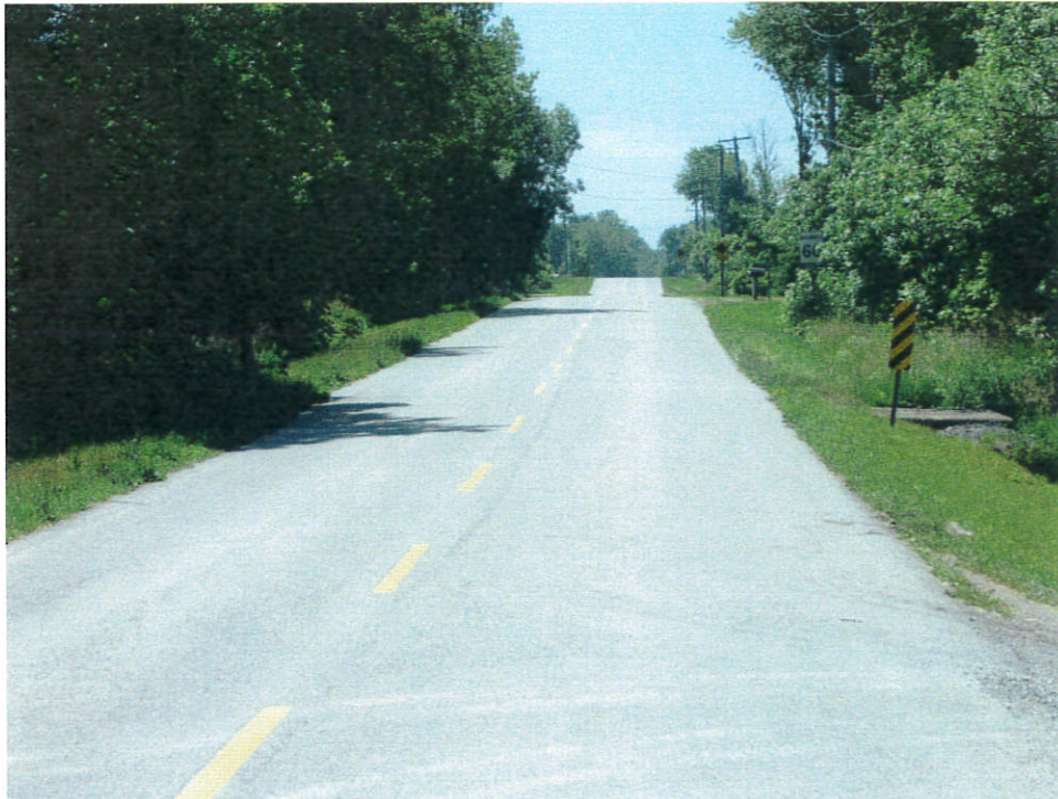
Roadway over the structure - Looking south
