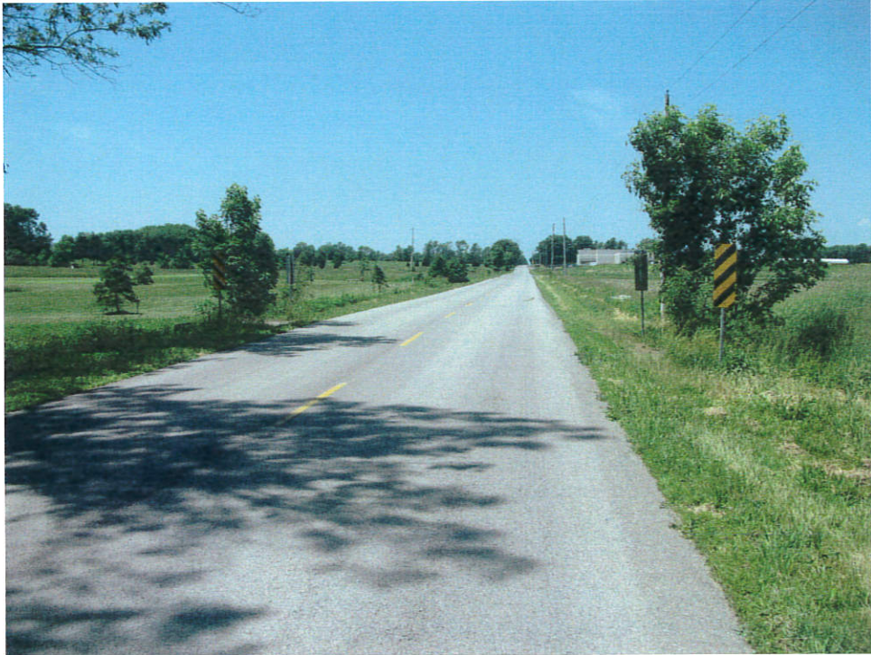
Roadway over the structure - Looking west
