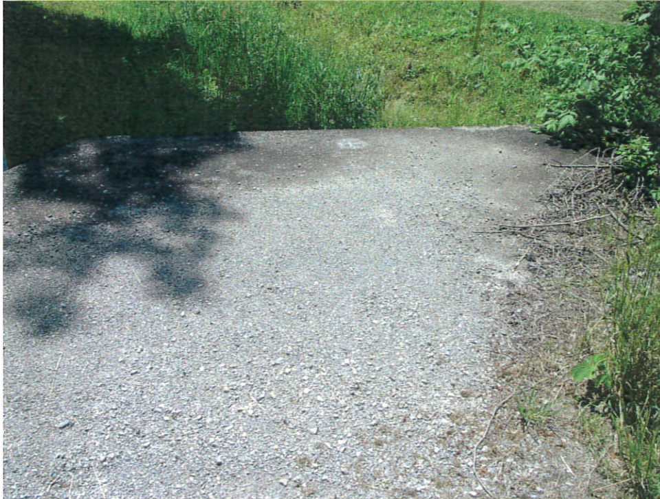
The south end of the structure
