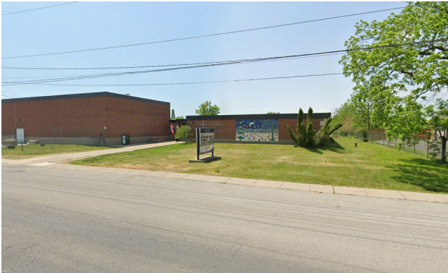
Image 2: Elementary School Catholic Saint-Joseph Source: Google Maps
